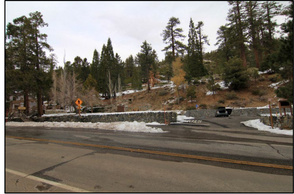
San Andreas Fault 1857 earthquake fault scarp forms steep slope at far end of parking lot.
