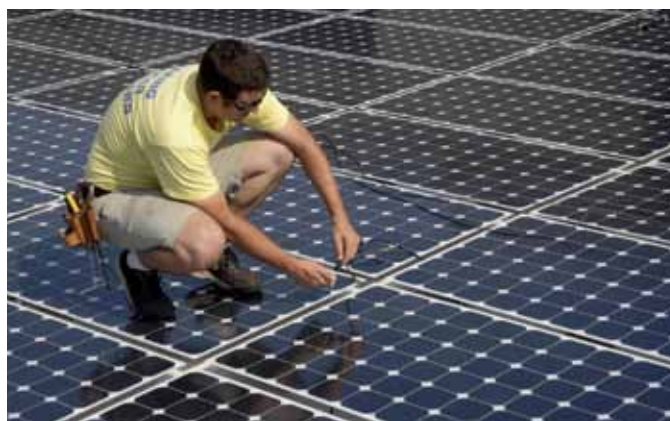
Illustration 8. Man wiring solar panels
