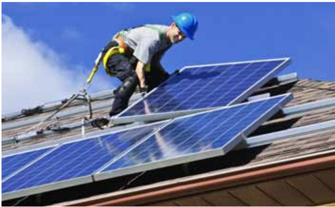
Illustration 10. Solar Photovoltaic installer with safety gear
