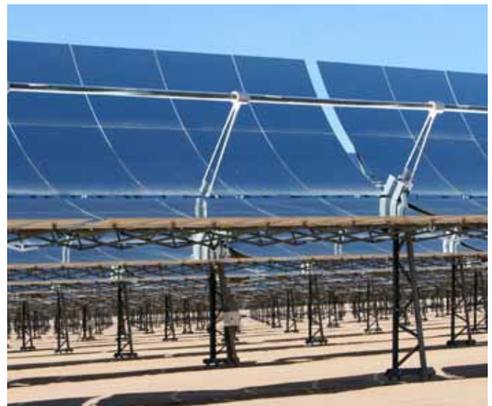
Illustration 3. Parabolic trough solar concentrators
