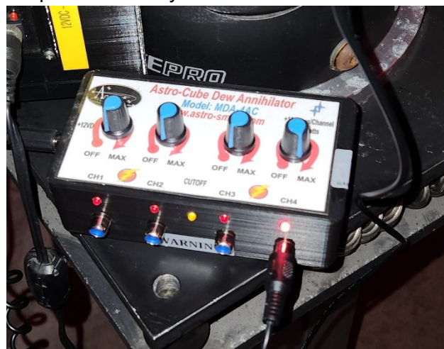
Figure 68 - Dew heater controller for the C14. Only one heating band is on the scope, so that is the only power source that is on.
